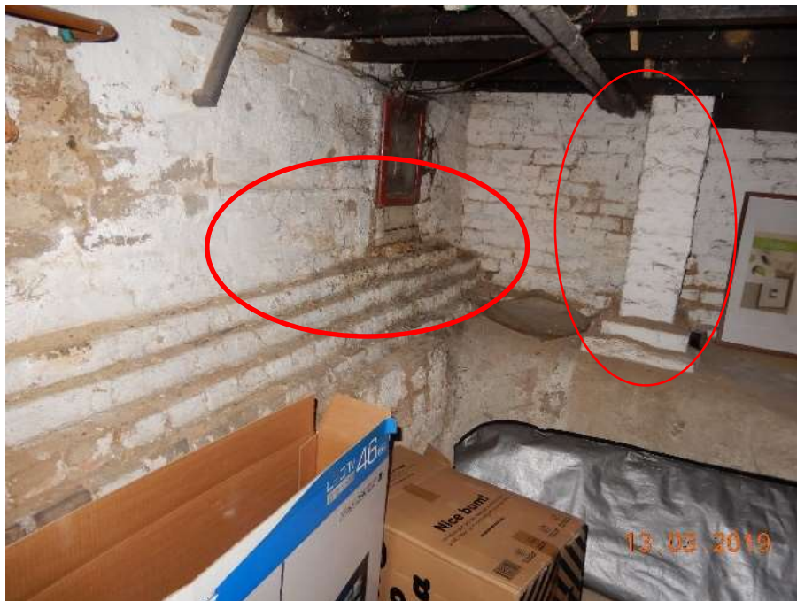
Figure No 26 Stepped brick spreader and pier foundation forming basement wall
