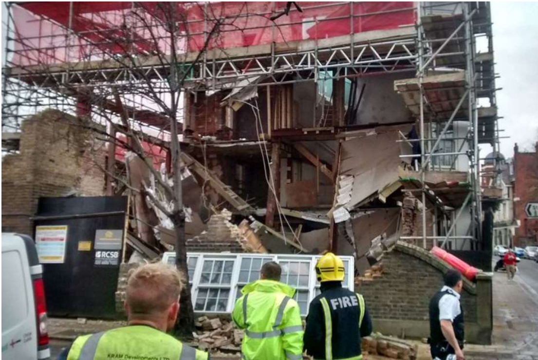
Figure No 3 Structural damage caused by botched basement construction (Evening Standard, 2015)
